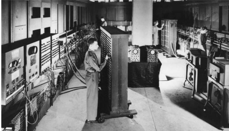
FIGURE E1.13.1 ENIAC, the world's first general-purpose electronic computer.
